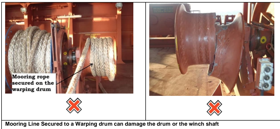
Fig 12: Mooring Winch Line secured to warping drum.
